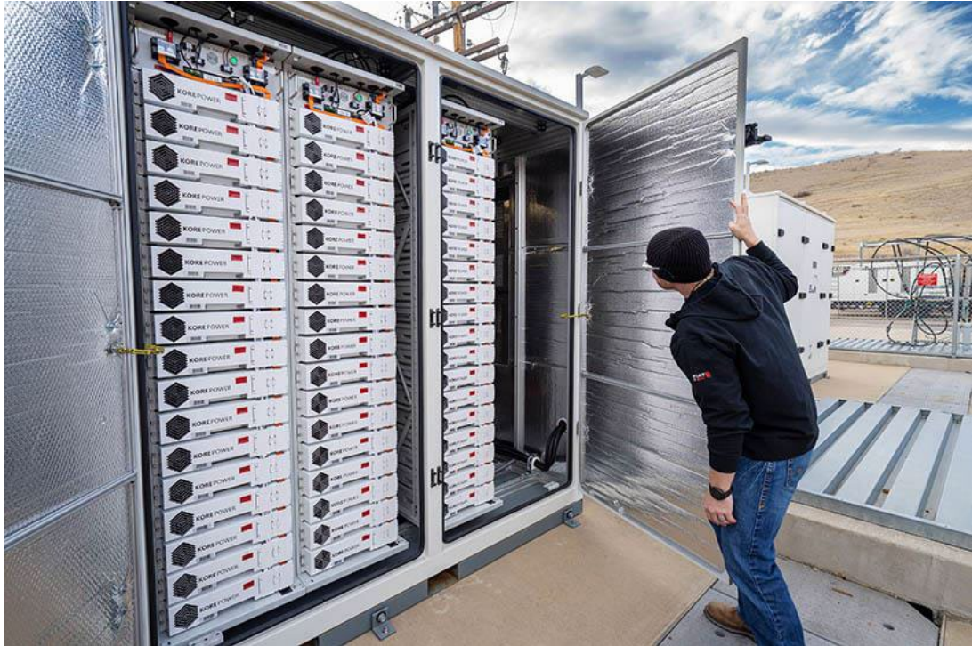
Plate 1-5: BESS access from the outside (Source: NREL)
